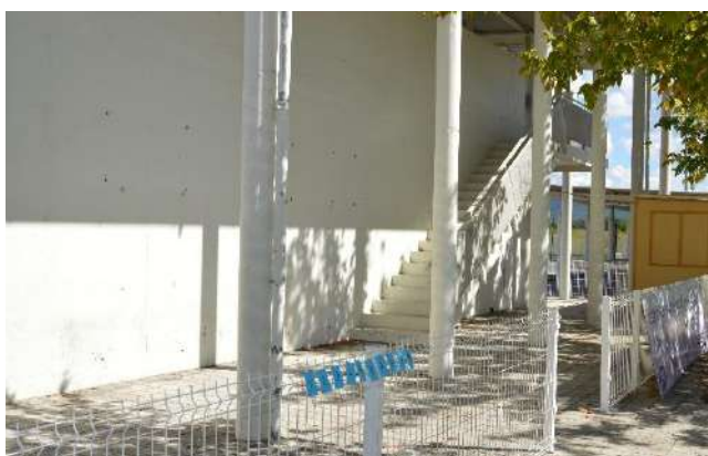
Driving stand stairs
